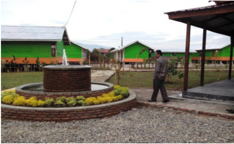
Picture 9: Integrated Community Shelter in Aceh
